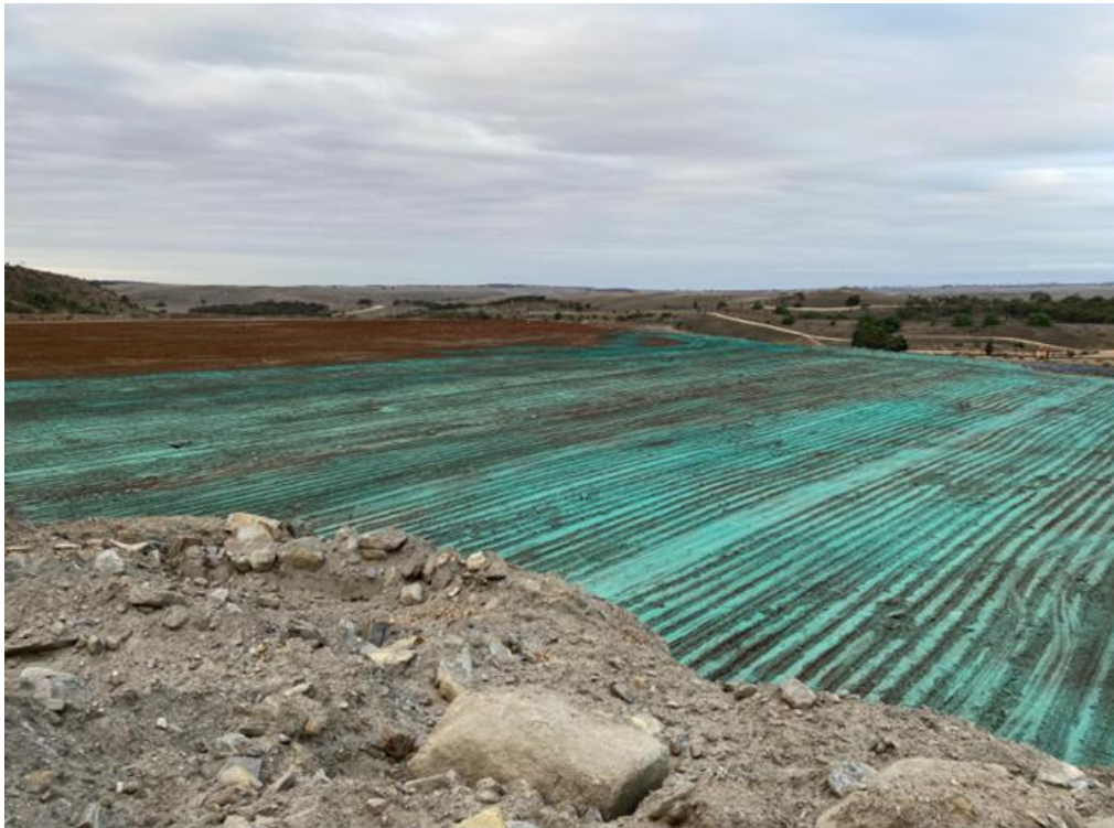
FIGURE 3. SEEDING OF THE REHABILITATED STOCKPILE AREA
